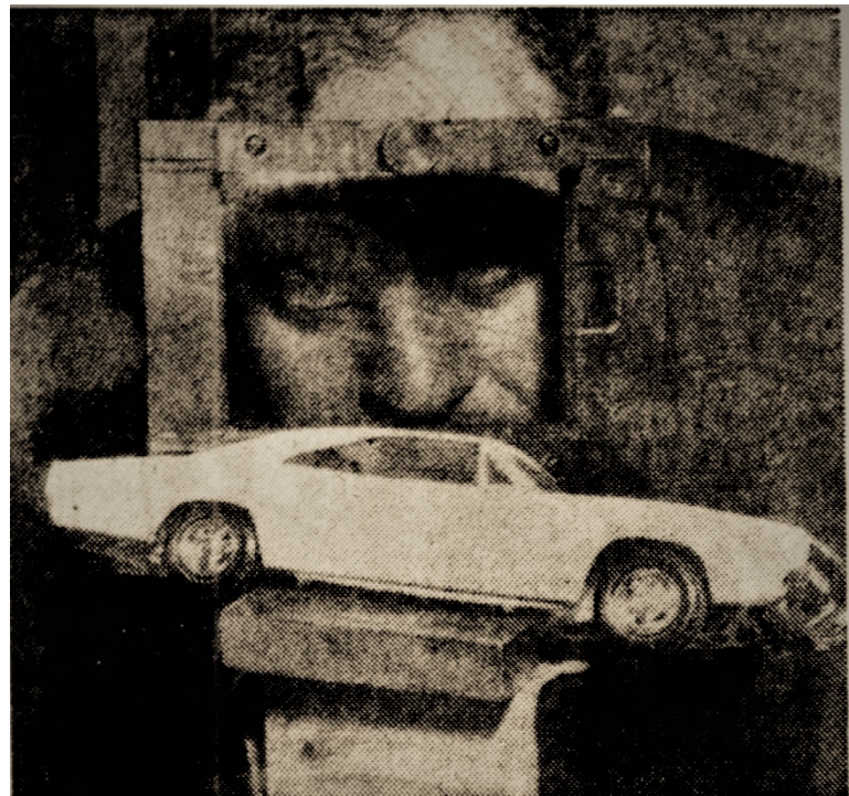
NEW CONCEPT —Dr. Joseph D. Hovanesian, Wayne State University engineering professor, peers through a photographic plate which when exposed to a Laser beam produces a three-dimensional figure. He says the auto industry could use this concept to test strains and pressures, and do it before a factory test car is built. (UPI Telephoto)
