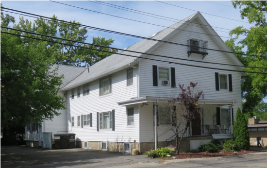
← House #10 Old Baptist Church, 4646 Moore St.
